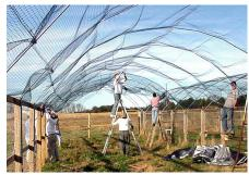
Hoops were bent and fastened into place and the aviary mesh roof went up. Gates were mass-produced. The finished product was a fully equipped, 2,000 square foot playground ready for running, climbing, and playing. Each cat run is 100 feet long (long enough to get up to a full speed run), 20 feet wide (plenty of room to zoom) and 12 feet high (for lots of climbing space). These runs would last through many snow and ice storms.
